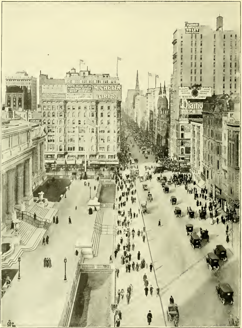
FIFTH AVENUE—North from 40th Street, formerly the center of fashion, is now a congested retail district, the corner of 42nd Street being the very heart of the famous White Light region. The Public Library extends for two blocks on the west side of the street.
